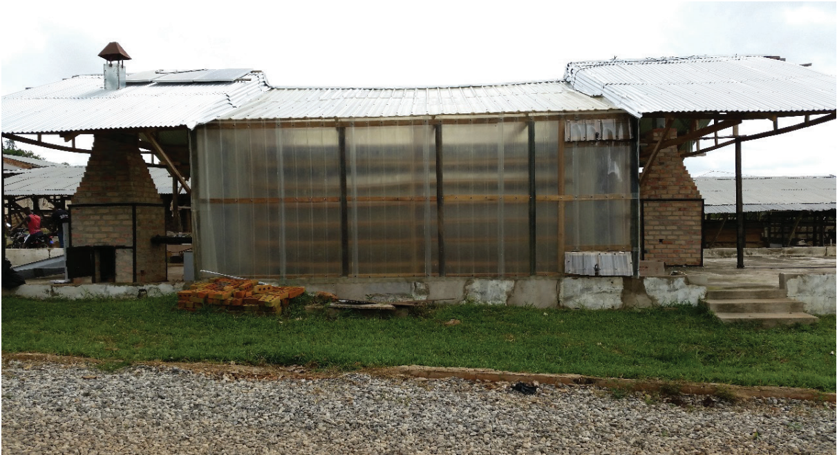
Solar Biomass Hybrid Dryer (SBHD) built by AMPLIFIES Ghana Project (KNUST) at Agona-Jamasi
